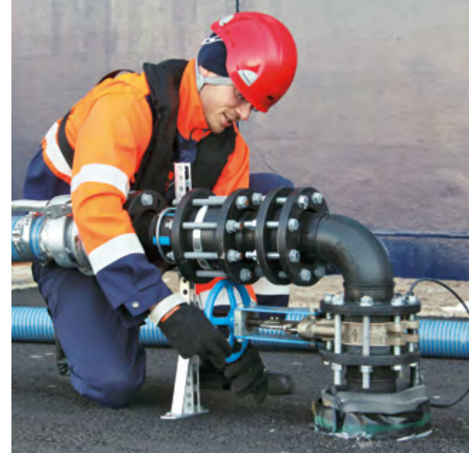
Each quay of the Port of Helsinki is equipped with a wastewater reception system for ship waste waters.
