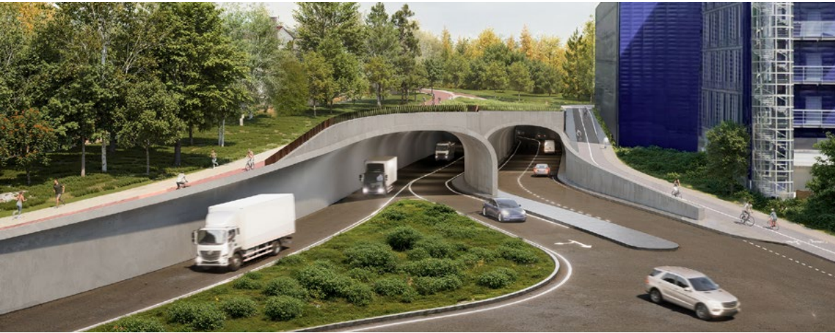
The West Harbour Tunnel's entrance on the Länsiväylä side has a concrete roof. Visualisation: PES-Architects Ltd.
